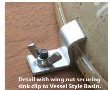
Vessel Style Sink secured to the under side of a mahogany counter with six sink clips fastened with wing nuts to 1/4 - 20 studs. Silicone adhesive additionally bonds and seals the sink rim to the carefully waterproofed wooden counter top.
